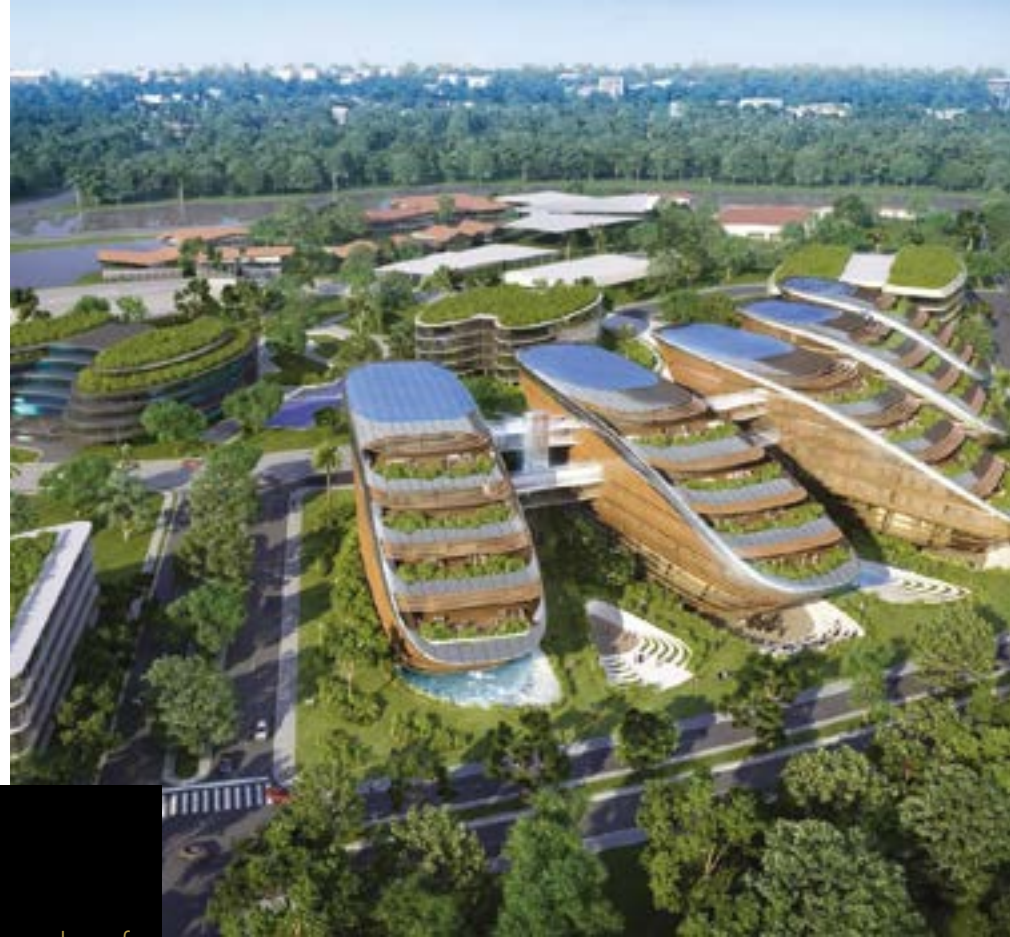
Green Office Park Development 05, Tangerang
