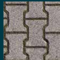
INTERNAL ROADS INTERLOCKING BLOCKS/ TREMIX CONCRETE ROAD
