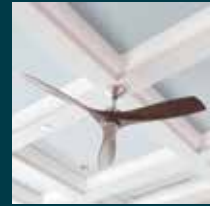
CEILING ACRYLIC EMULSION PAINT/ OIL BOUND DISTEMPER
